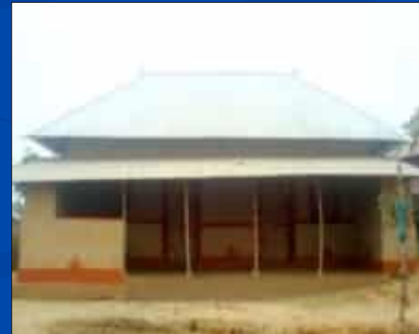
Completed earthen house
